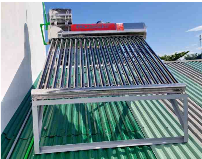
Solar hot water unit on the roof.
