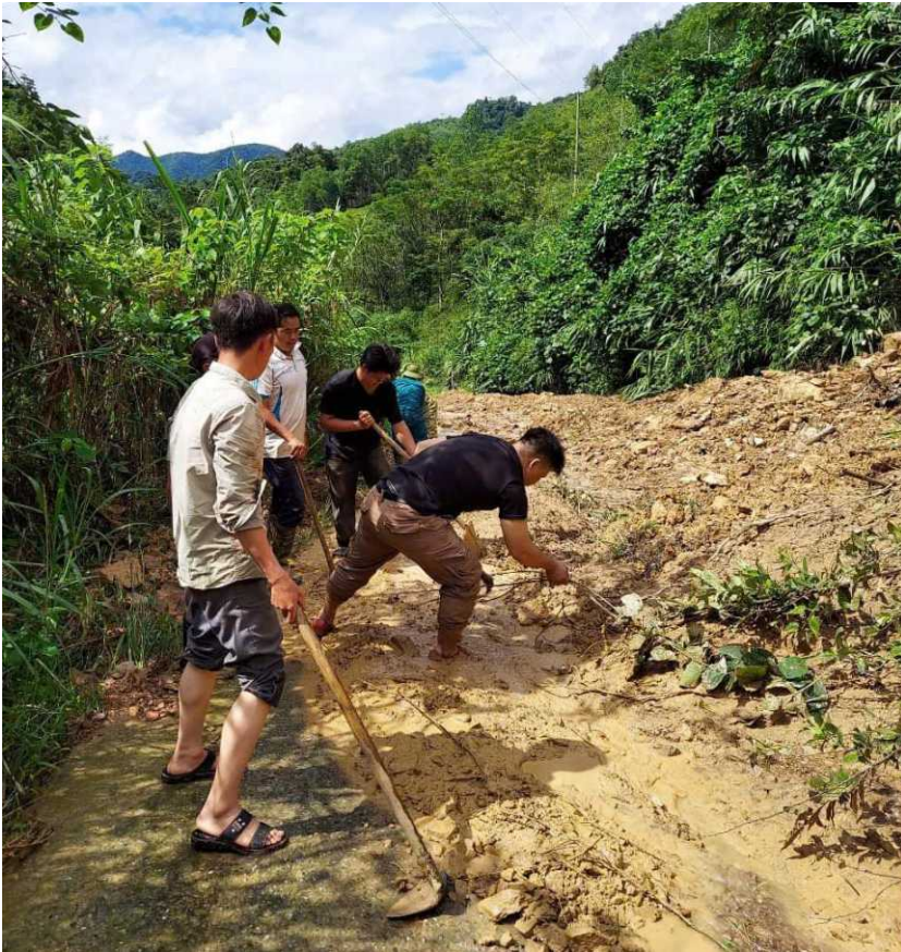
Clearing a soil slide to make the track passable
